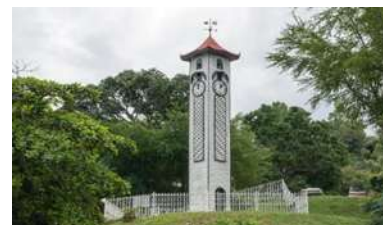
Figure 14. Atkinson Clock Tower
